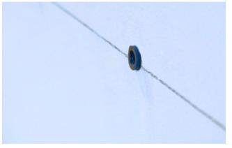
**Step 6:** Screw the knob onto the screw, then insert the knob and screw through the sheet and screw clockwise into the anchor.
